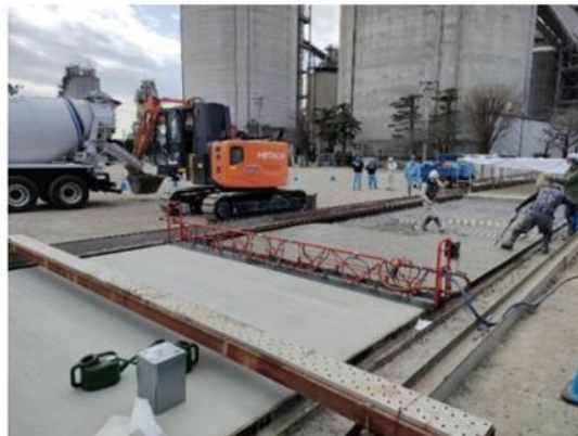
Photo 4. Test construction of pavement concrete using CARBOCATCH slurry
