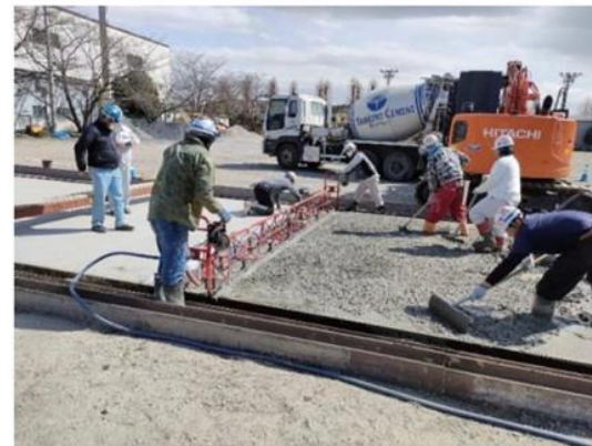
Photo 4. Test construction of pavement concrete using CARBOCATCH slurry
