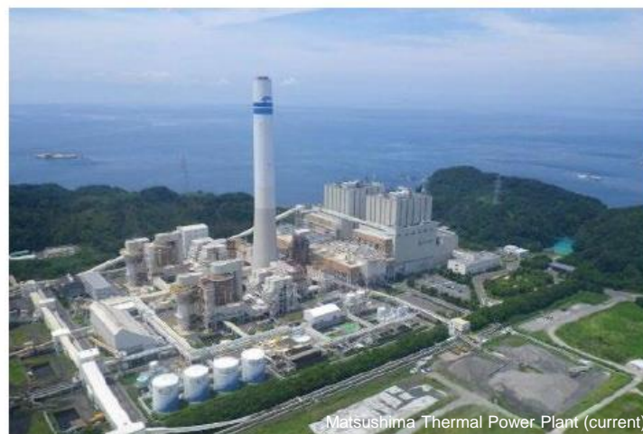
Matsushima Thermal Power Plant (current)
