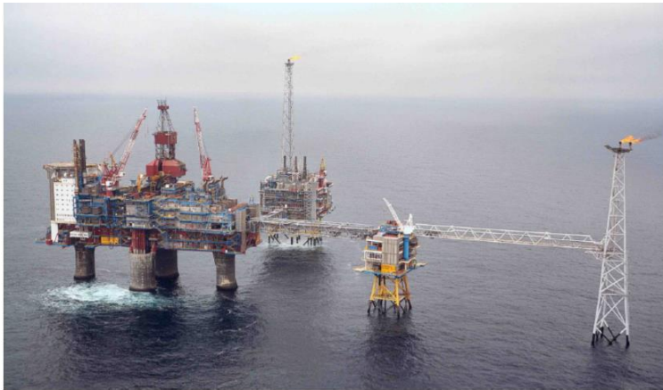
The world's first and longest lasting commercial storage project (since 1996, 20+ Mt CO 2 stored).
