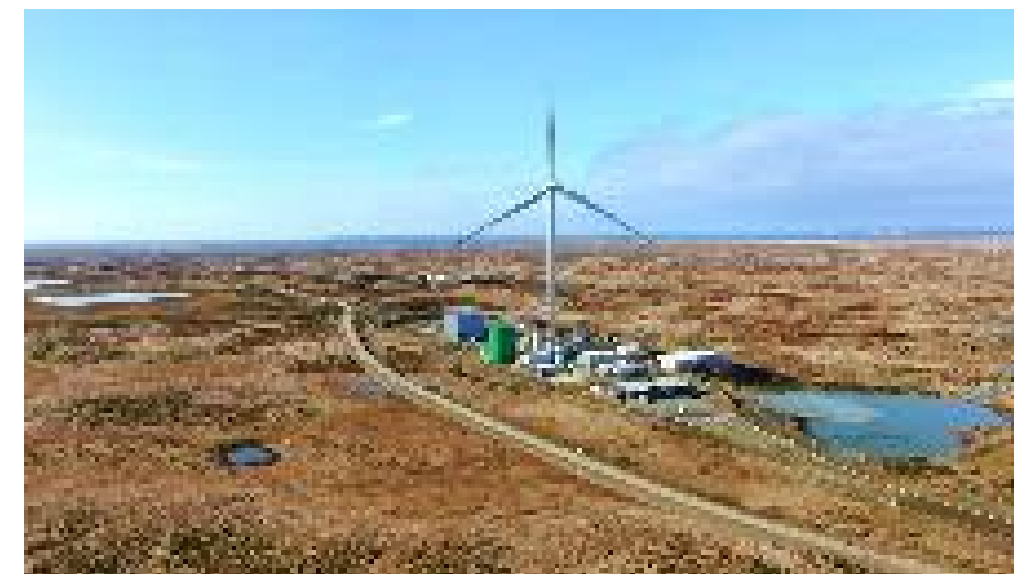
HIF Global LLC operates the world's first operational e-fuels plant from 2022, Haru Oni, Chile.
